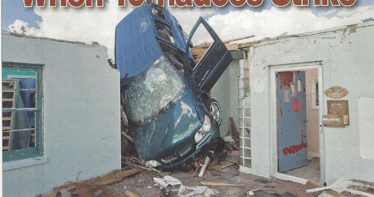
▲ A powerful tornado in Kansas threw this van against a hotel building.
