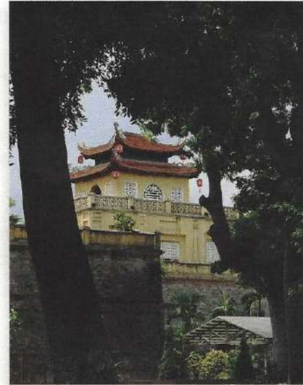
The newly restored pavilion inside the former imperial citadel of Thang Long in Hanoi, Vietnam
