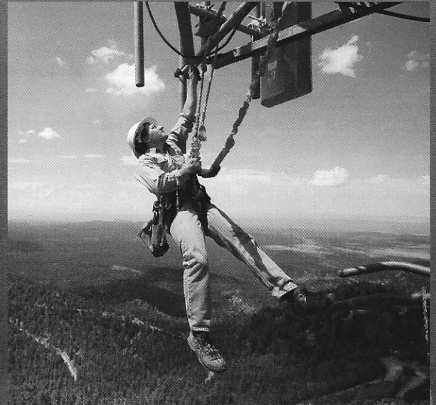
▲ A repair person working on a radio tower
