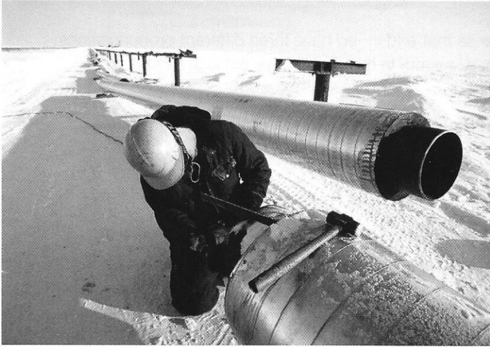
▲ Working on oil pipes in Alaska
